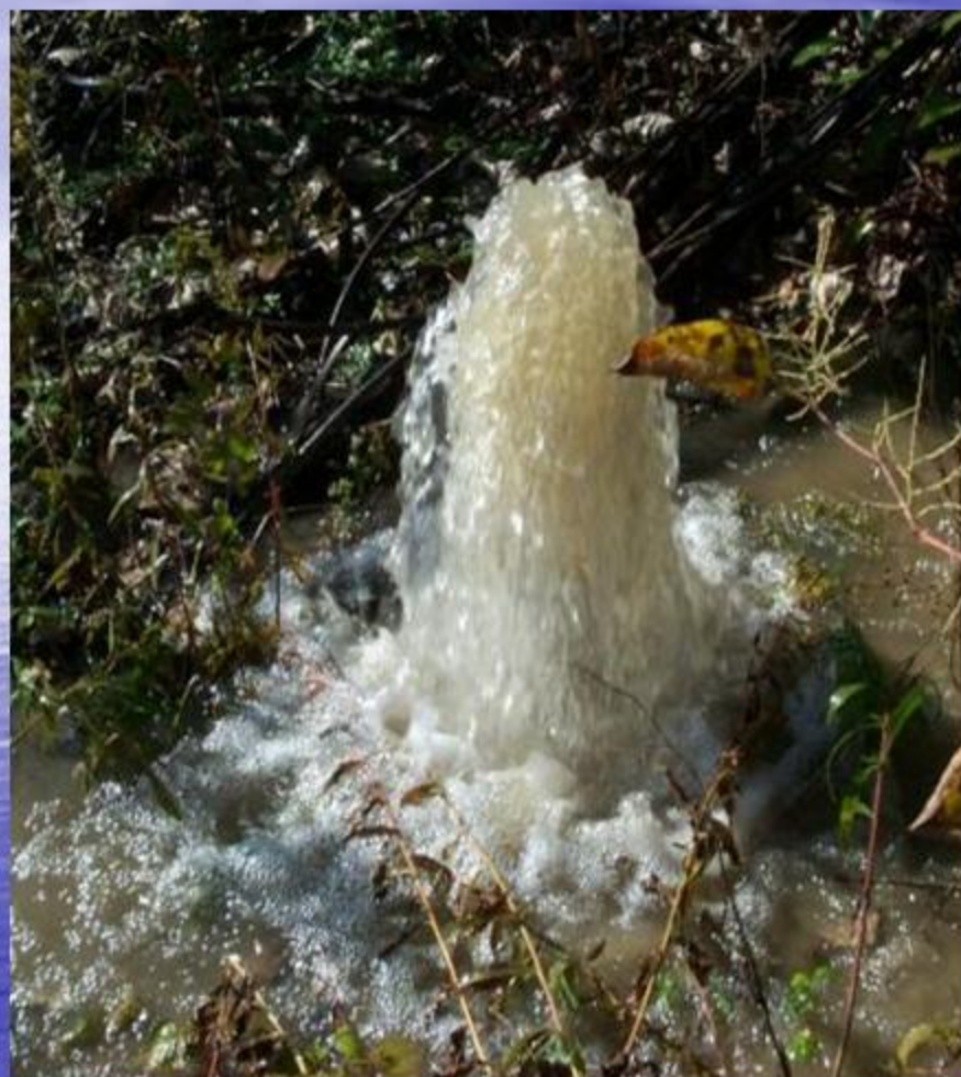
Groundwater response to grout injection
